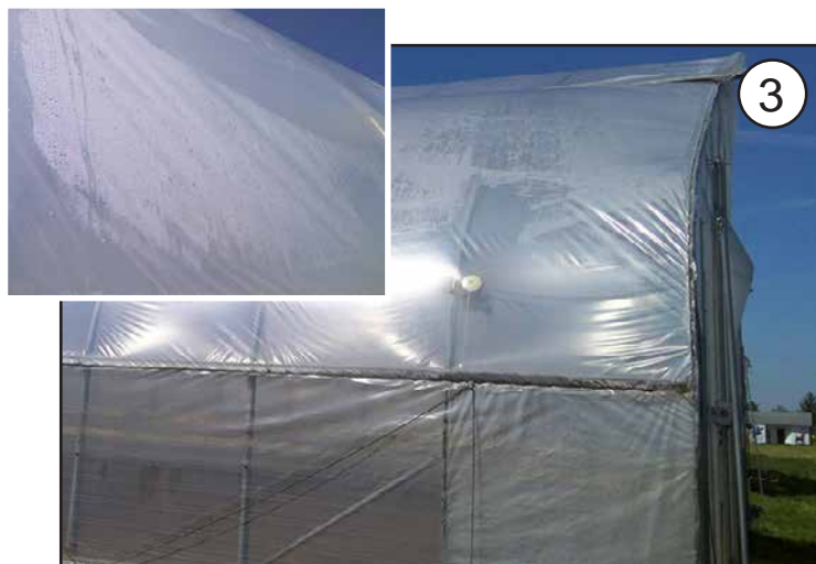
FIGURE 3. WHEN EXCESS WATER VAPOR IN THE AIR IS RELEASED, IT CAN RESULT IN CONDENSATION ON HIGH TUNNEL SIDEWALLS. NOTE THE INSET SHOWING A CLOSE-UP OF CONDENSATION.
